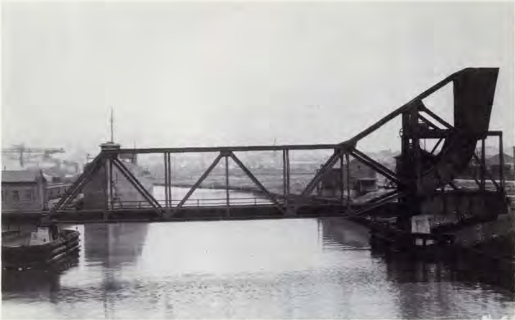
Scherzer Rolling Lift bridge over the Cuyahoga River, built for the B&O Railroad.
