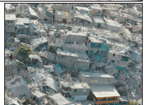
TOP: Vadim Levtonyuk (standing to the left, wearing an orange shirt, dark vest, and pants) and his companions wait to leave Port-au-Prince airport. BOTTOM: Dozens of the thousands of buildings that collapsed in Port-au-Prince. Photos courtesy of Slavic Full Gospel School.
