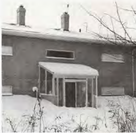
North entry (back of house) has glazed foyer to prevent heat loss.
