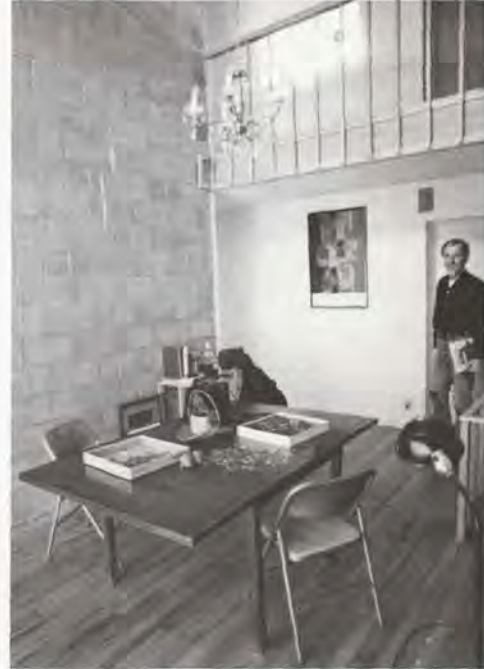
Floors and balcony use wood from oak trees cut from building site.
