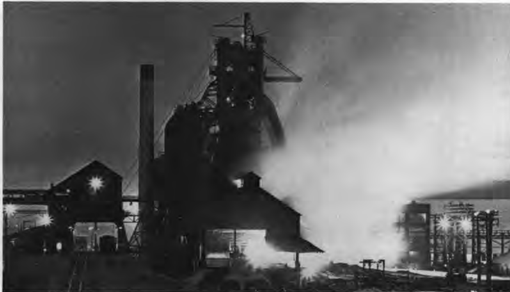
Though the predominant means of making steel since the late 1800s, the blast furnace has become an American dinosaur. Pictured above is one of the remaining American blast furnaces in operation.
