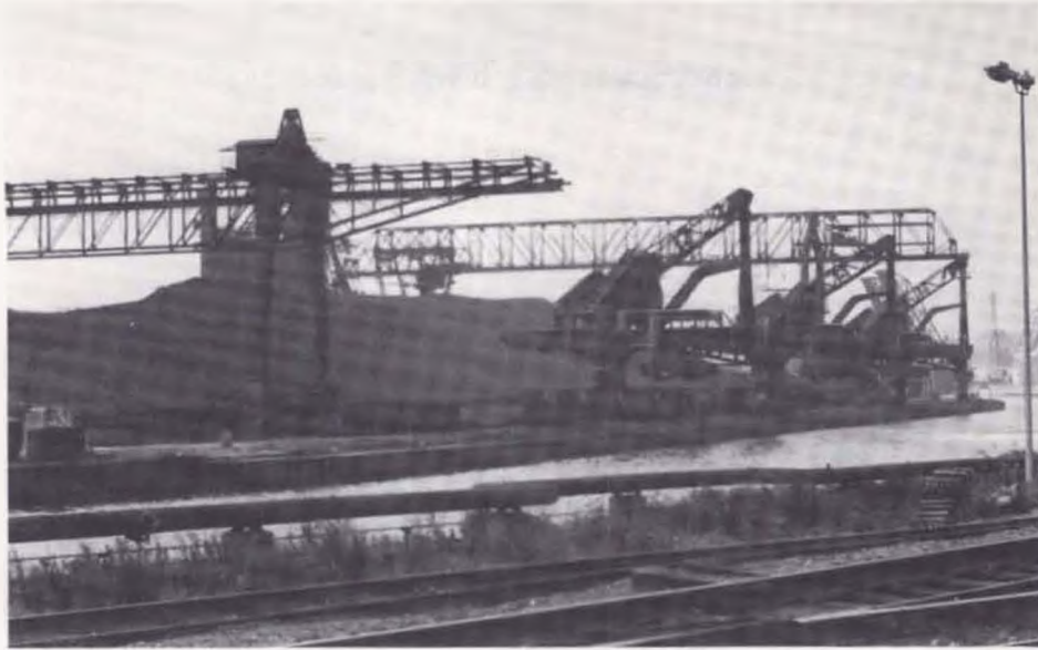
Corrigan, McKinney and Company Ore Dock, (1910-1916)
