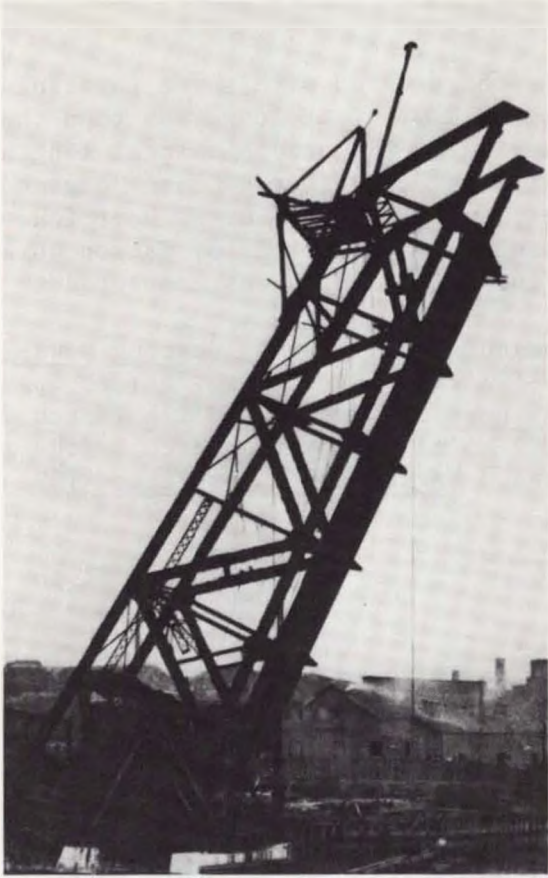
Newburgh and South Shore Railroad Bridge, (1904)
