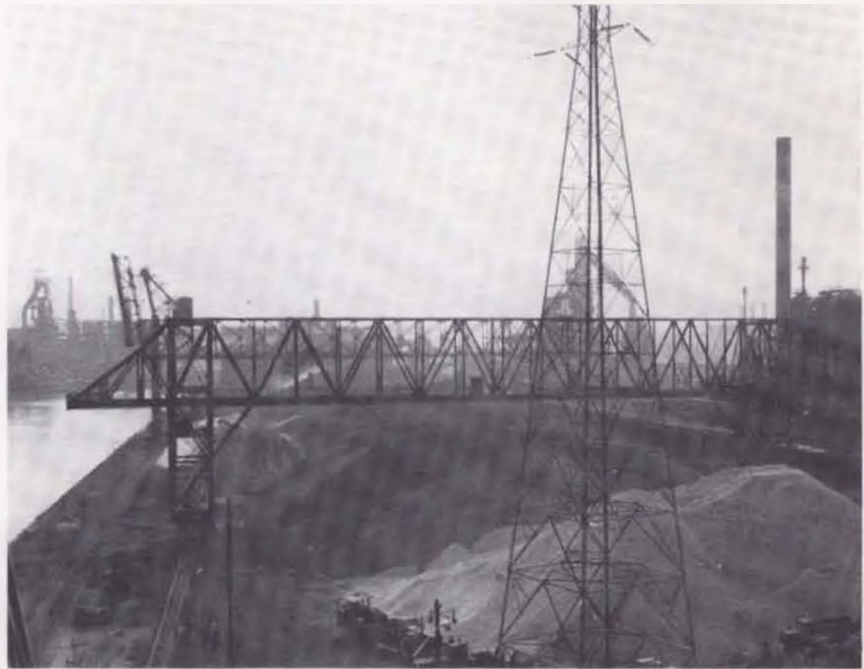
Otis Steel Company Ore Dock, (1913-1914); 1919 Ore Handling Bridge Operates Over Self-Unloading Dock
