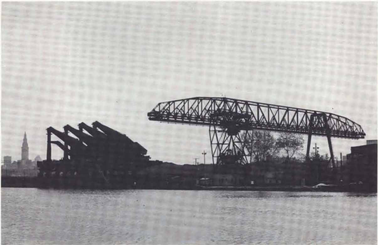
Pennsylvania Railway Ore Dock, (1912)
