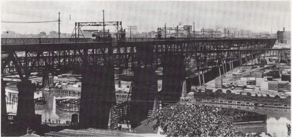
Central Viaduct, River Section, (1878), New York, Chicago and St. Louis Railroad Viaduct runs underneath
