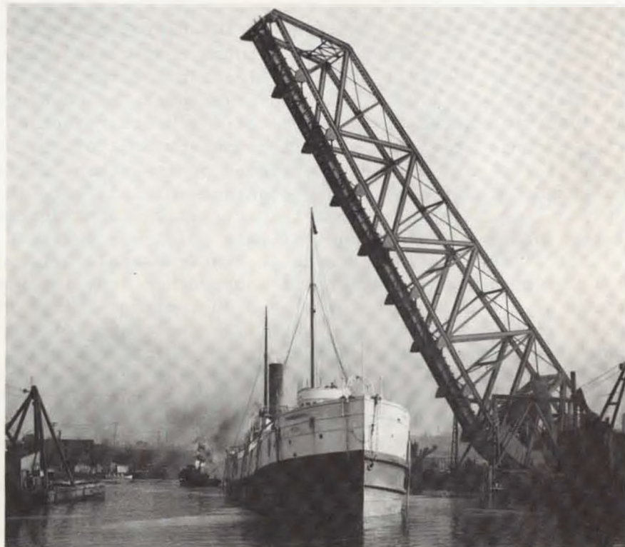
Lake Erie and Wheeling Bridge, (1906) across Old River Bed
