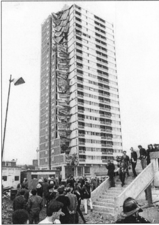
Fig. 1. Ronan Point after collapse
