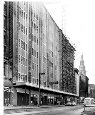
Taylor Department Store Renovations, 1966
