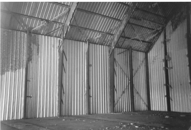
Fig. 2. Warehouse interior framing
