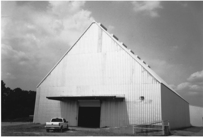
Fig. 1. Exterior view of warehouse
