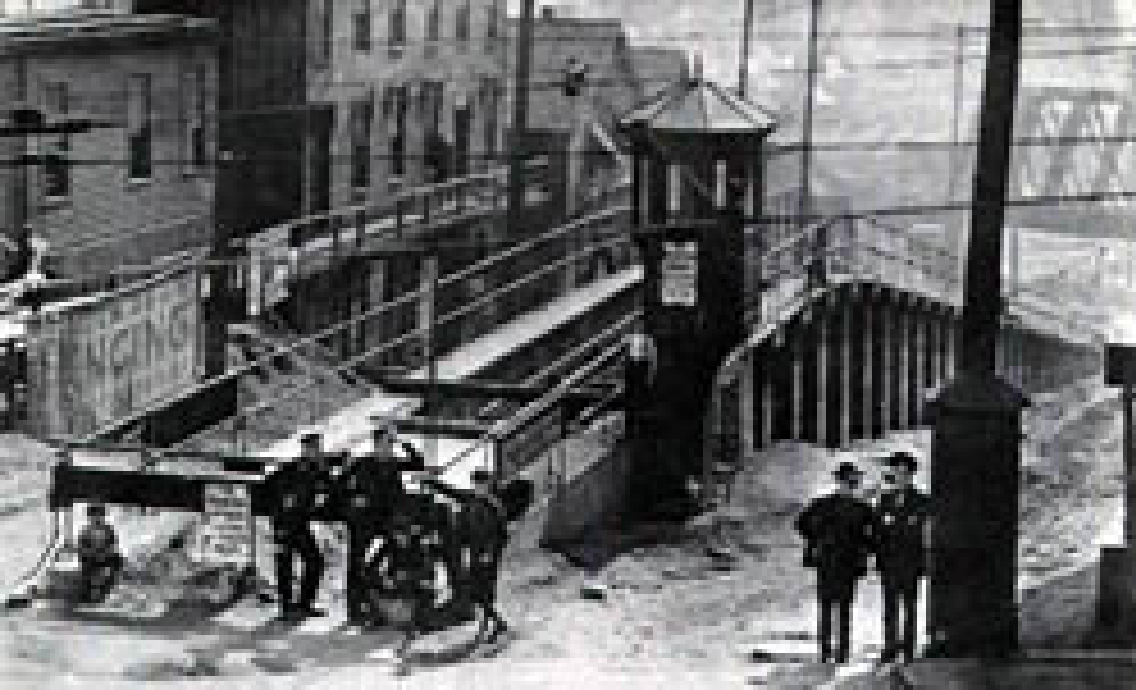
The Rolling Road under construction – circa 1905 Courtesy of the Plain Dealer, Cleveland, Ohio
