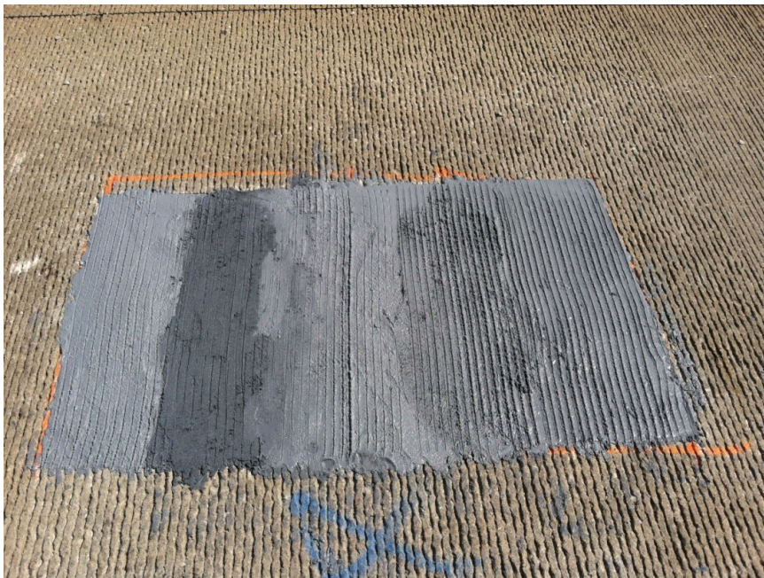
Figure 27: Patch #36, containing Delpatch, showing a dark spot due to batch completed with improper material measurements.
