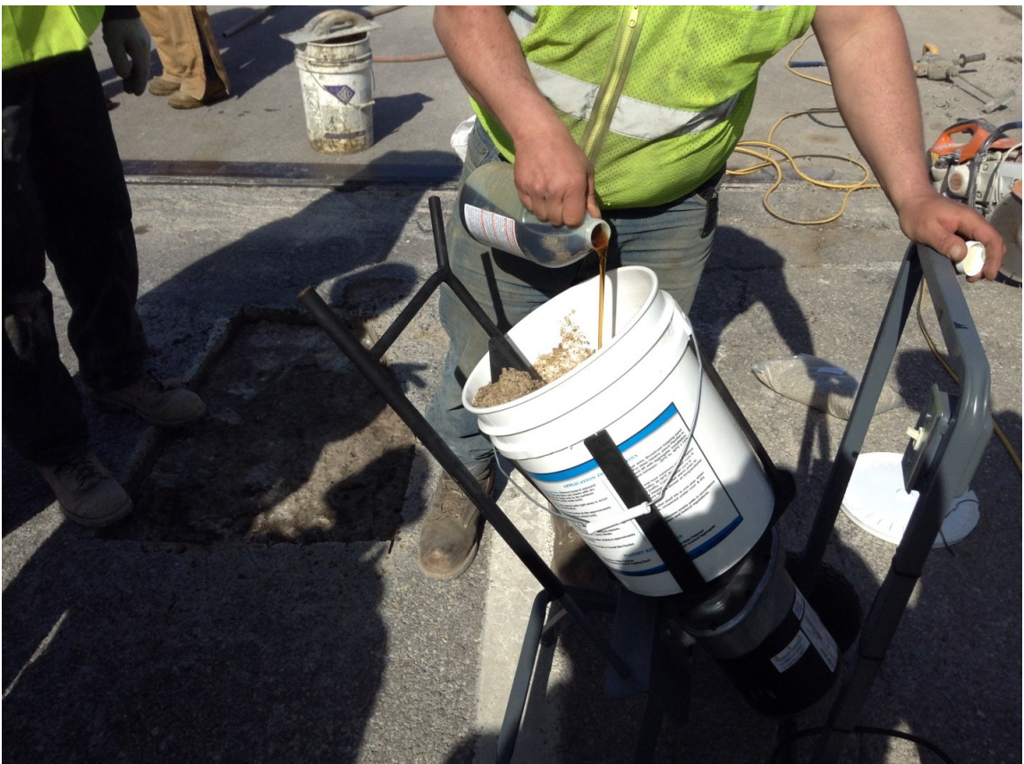
Figure 5: The Motor Mix Machine in use, which is a specialized mixer for the FlexSet product.
