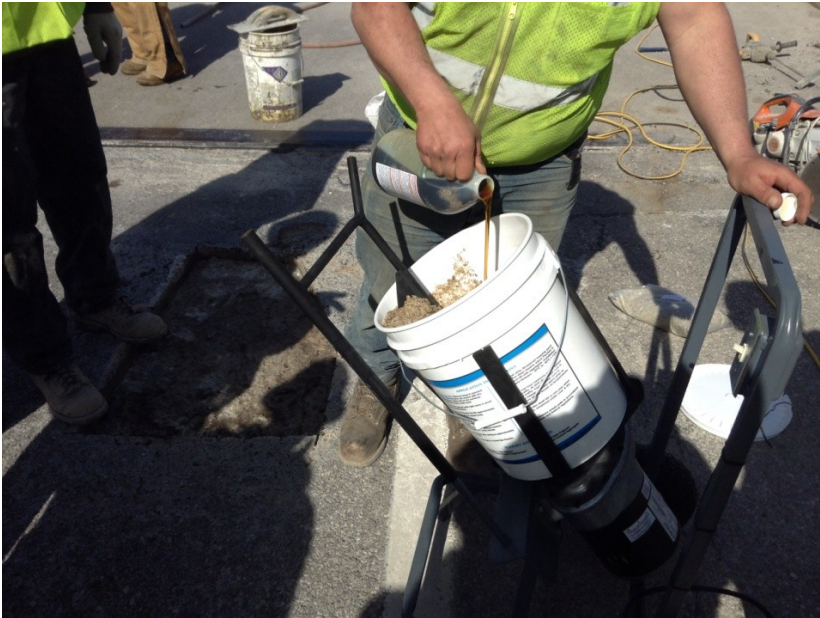
Figure 12: Mixing Flex Set patching material.
