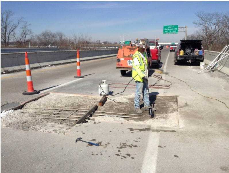
Figure 11: Drying the hole with a torch.
