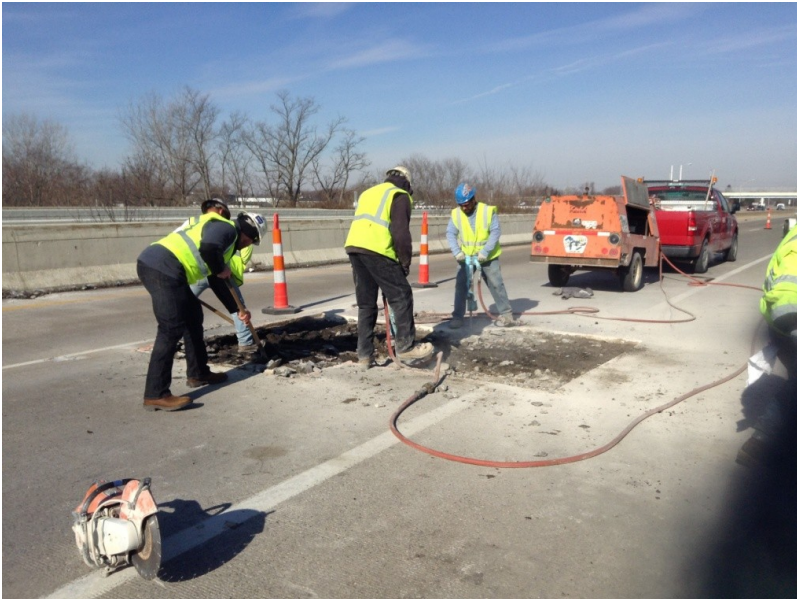
Figure 10: Removing the pavement with jackhammers.
