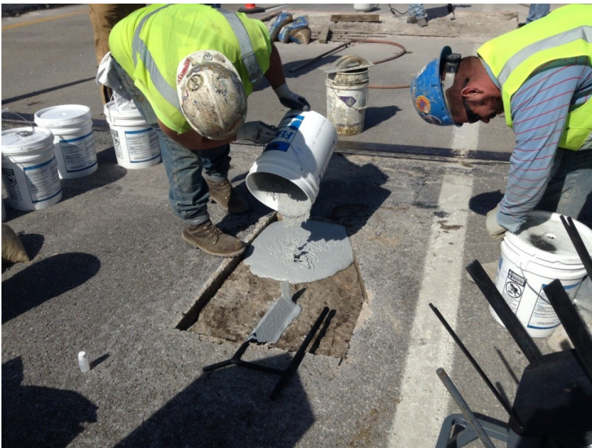
Figure 13: Filling hole with Flex Set patching material.
