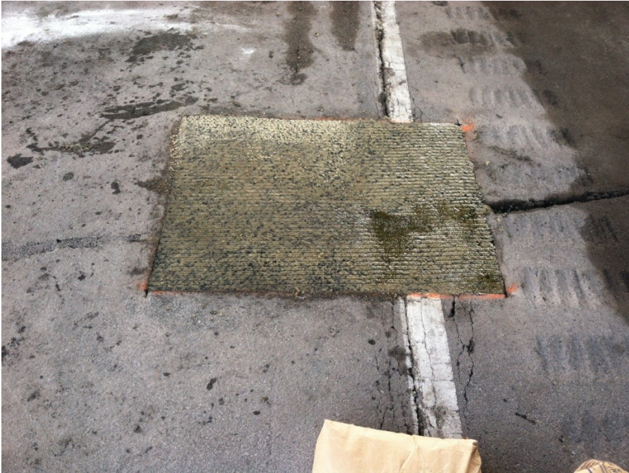
Figure 22: Patch #16, containing SR-2000, placed over an expansion joint.
