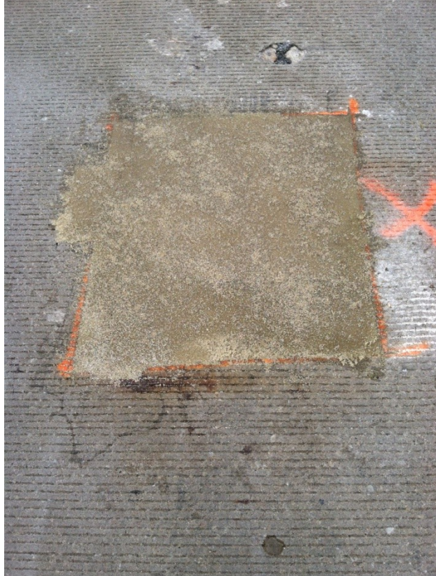
Figure 26: Patch #30, containing SR-2000, showing an extension (ear) on the middle left of the patch.
