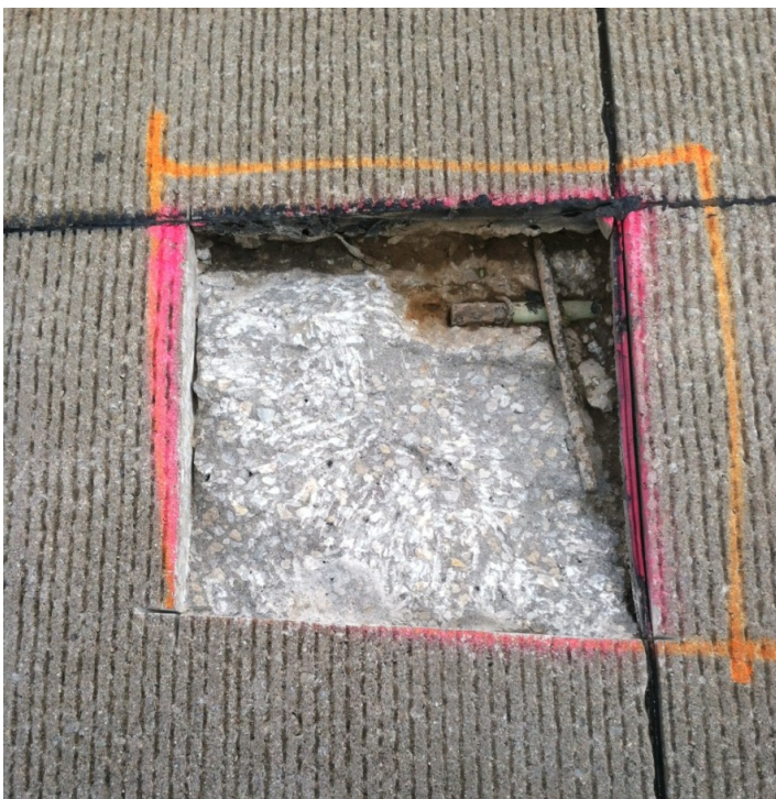
Figure 21: Patch #75, placed at an expansion joint.
