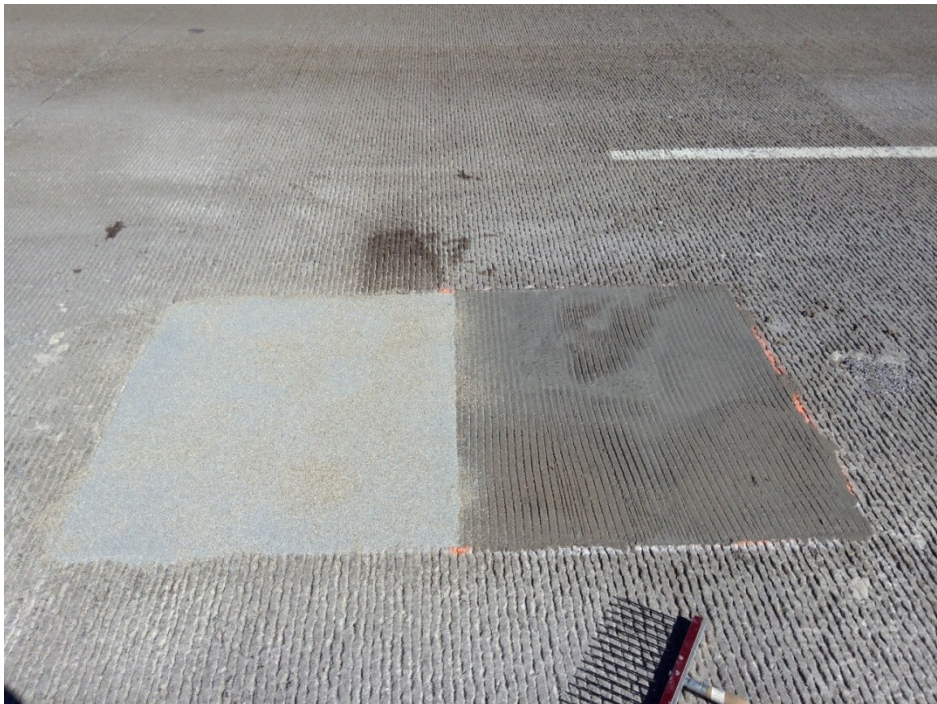
Figure 14: Patches #9 (left) and #10 (right), containing FlexSet and MG Krete, respectively.
