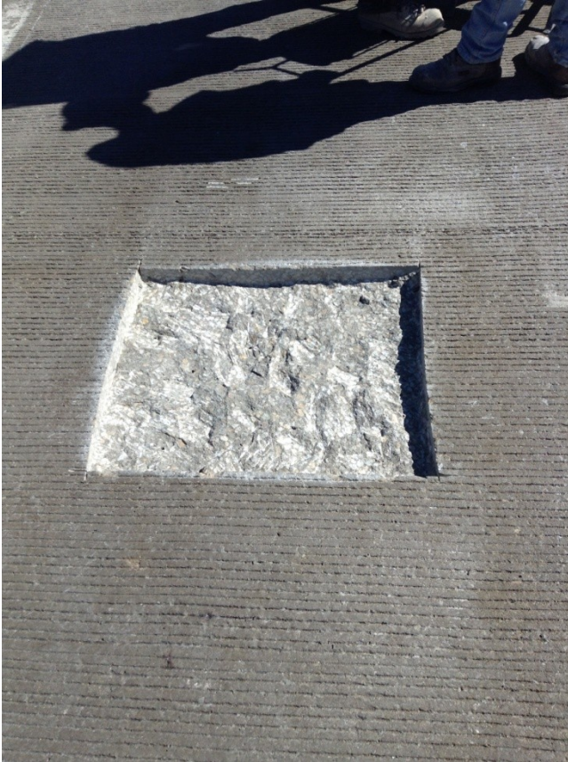
Figure 37: An example of a clean, smooth-cut hole, where patch #14 was installed.
