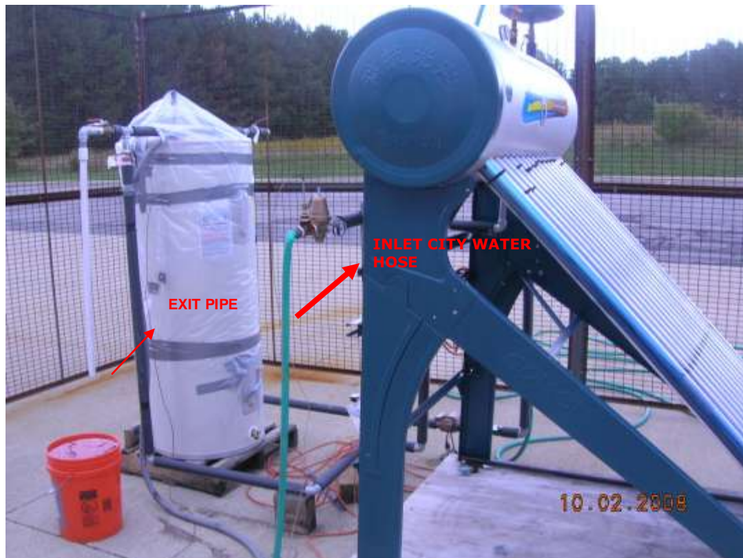
Figure 22: Solar Water Heater connected in series with the Hot Water Tank. Courtesy: [HMI Industries]
