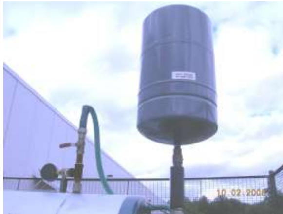
Figure 12: EXTROL Expansion Tank. Courtesy: [HMI Industries]
