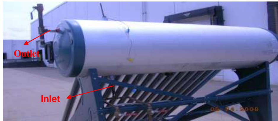
Figure 5: Location of Inlet and Outlet. Courtesy:[HMI Industries, Ohio]
