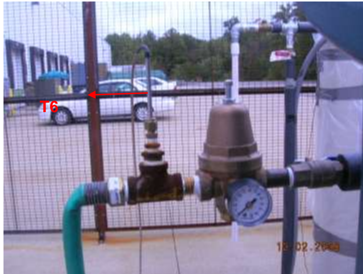
Figure 20: Pressure reducer and Thermocouple T6. Courtesy: [HMI Industries]
