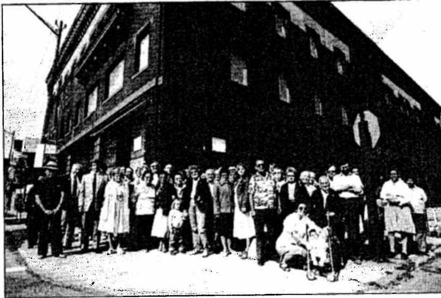
Area residents working with the Near West Housing Corporation in Cleveland, helped save the 18-unit Miller Building from the city's wrecking ball. A board of neighborhood residents will control the management of the building.
