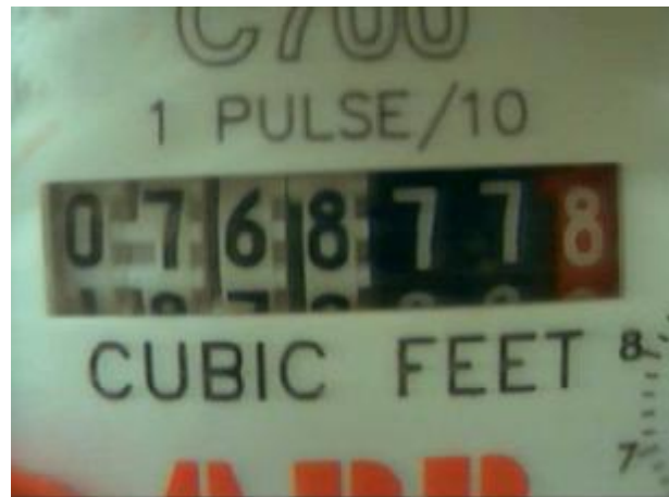
Figure 16 Original utility meter image #1
