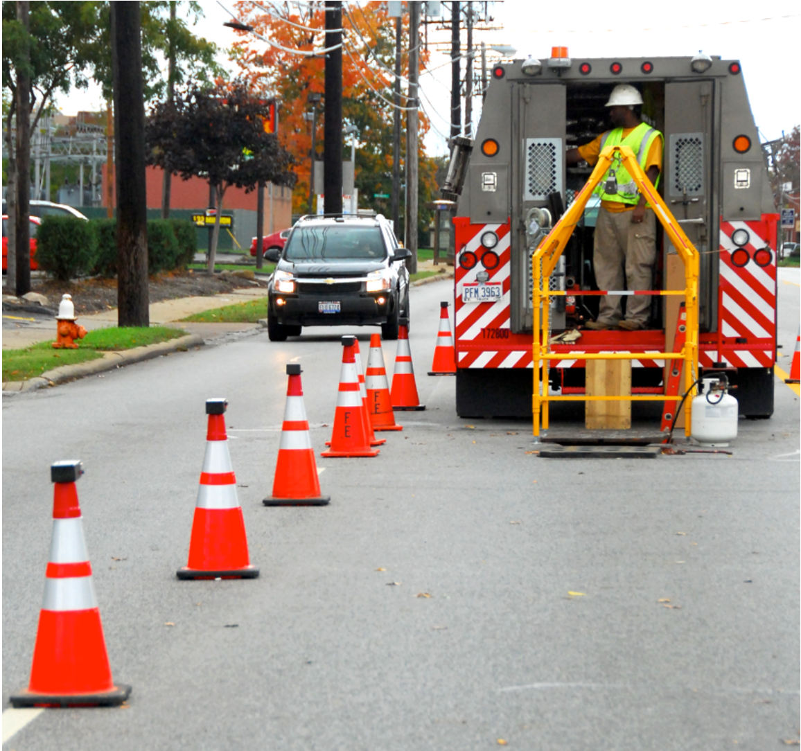
Figure 2: Our sensornet system deployed in a work zone to collect traffic statistics. The nodes are mounted on top of construction safety cones. The placement of the cones is as required by the work zone itself as per the MUTCD, and is not modified by our deployment.
