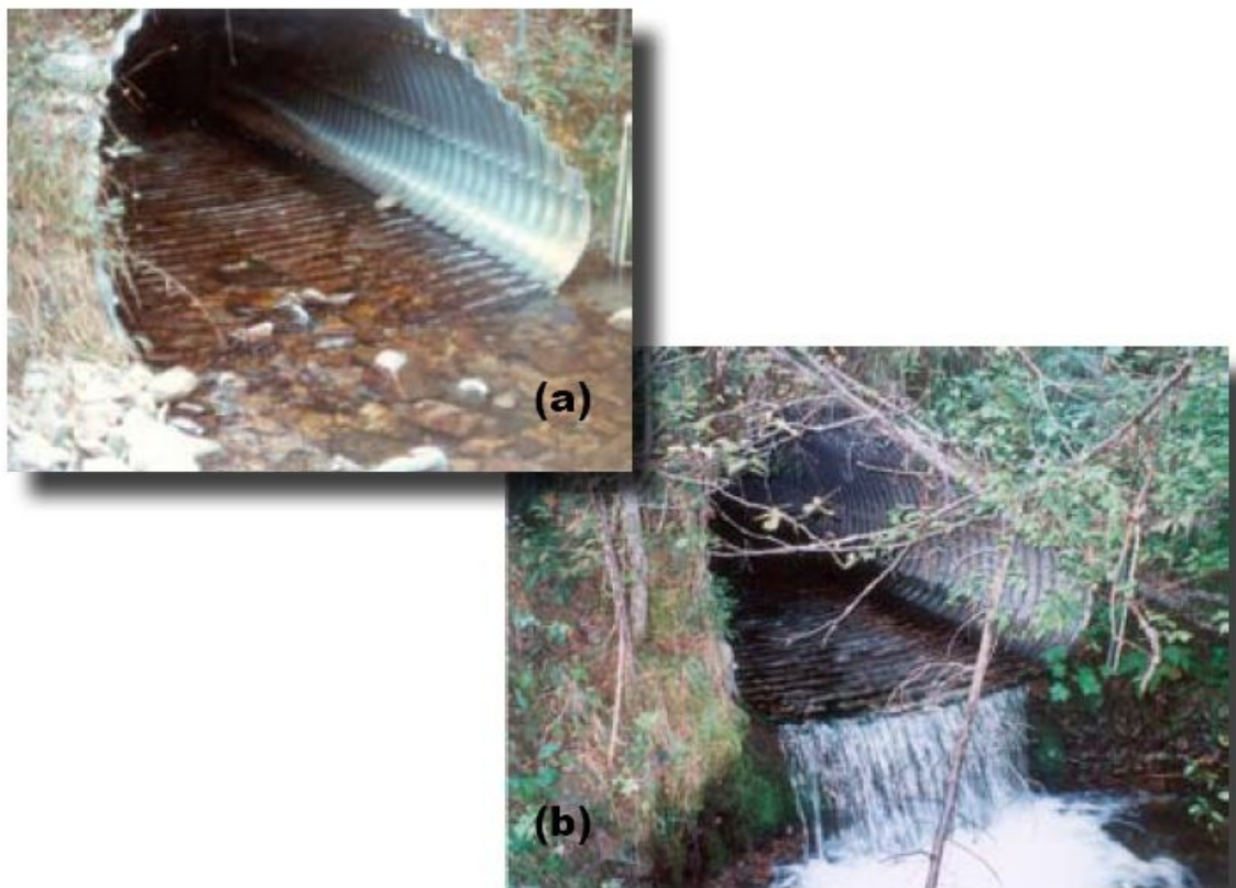
Figure 1.1 Perching of a Culvert as a Result of Long-Term Scouring (Forest Service Stream Simulation Working Group, 2008)
