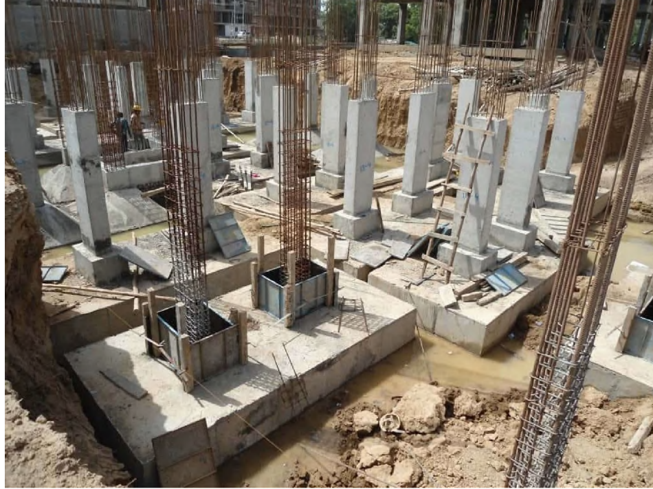
Figure 1. Rectangular combined footings [7].
